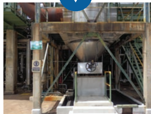
Steps widen, hand railing installed
