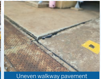
Uneven walkway pavement
