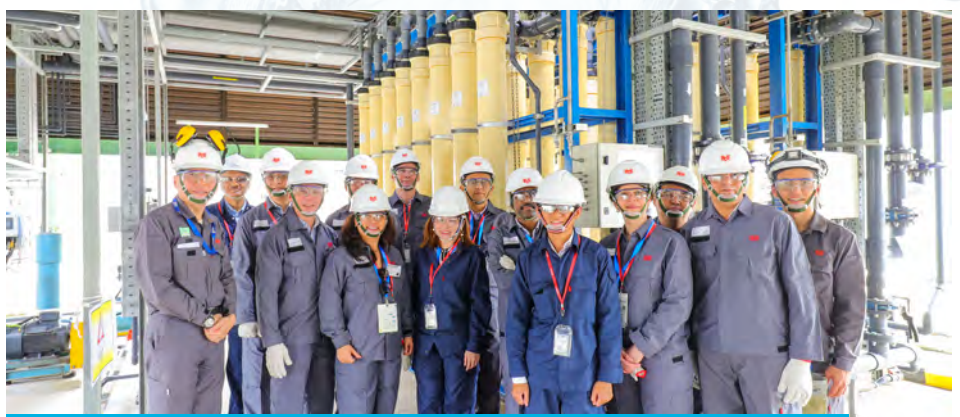
Delegates at Treated Wastewater Recovery Plant (pre-treatment MF) and Top (Left: RO modules, Right: Activated Carbon Filters).
