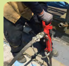
Photo after intervention with whip arrestor
