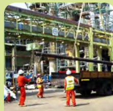
Photo after intervention, avoid working below object
