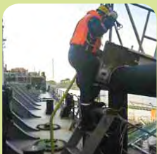
Photo after intervention with proper access ladder
