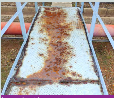
Corroded walkway platform
