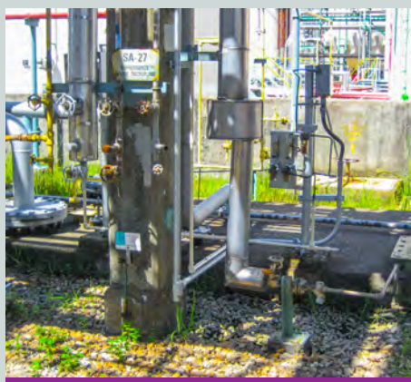
Damaged insulation rectified
