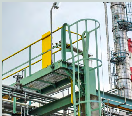
Installed metal backing to prevent valve key from dropping from height
