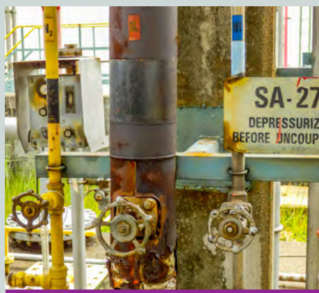
Damaged insulation - scalding risk
