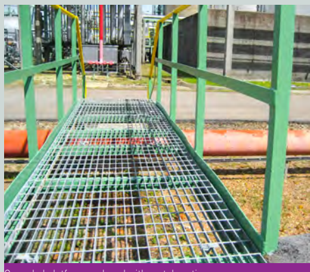
Corroded platform replaced with metal grating
