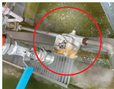
Picture from Techmatic: Example of faulty steam trap (circled)
